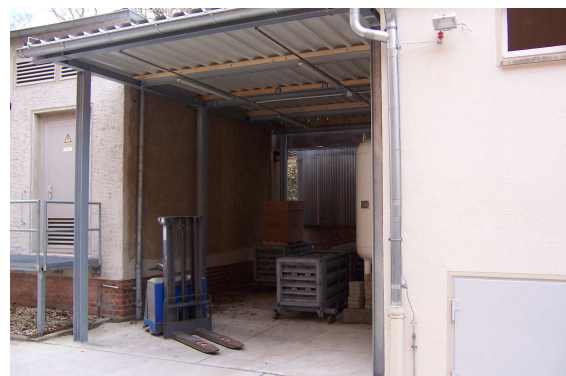
Fig. 2: Adverse weather cover for the storage area of the He-gas transport units
