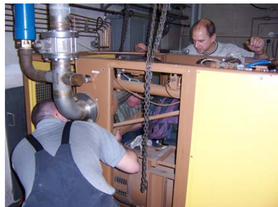
Fig. 3: The main He-compressor under repair
